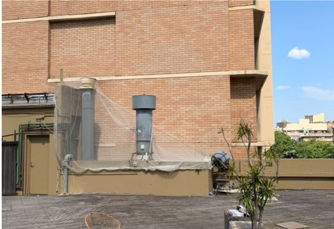
view from rooftop looking south east
