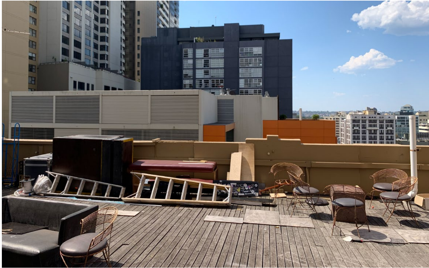
view from rooftop looking north
